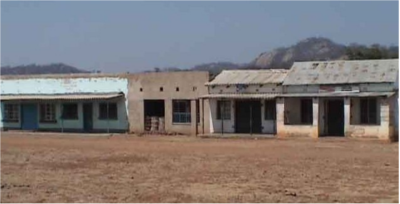
Photo 6: rural business centre in Matabeleland entirely closed after price slashes emptied shelves and made restocking financially impossible. August 2007.
