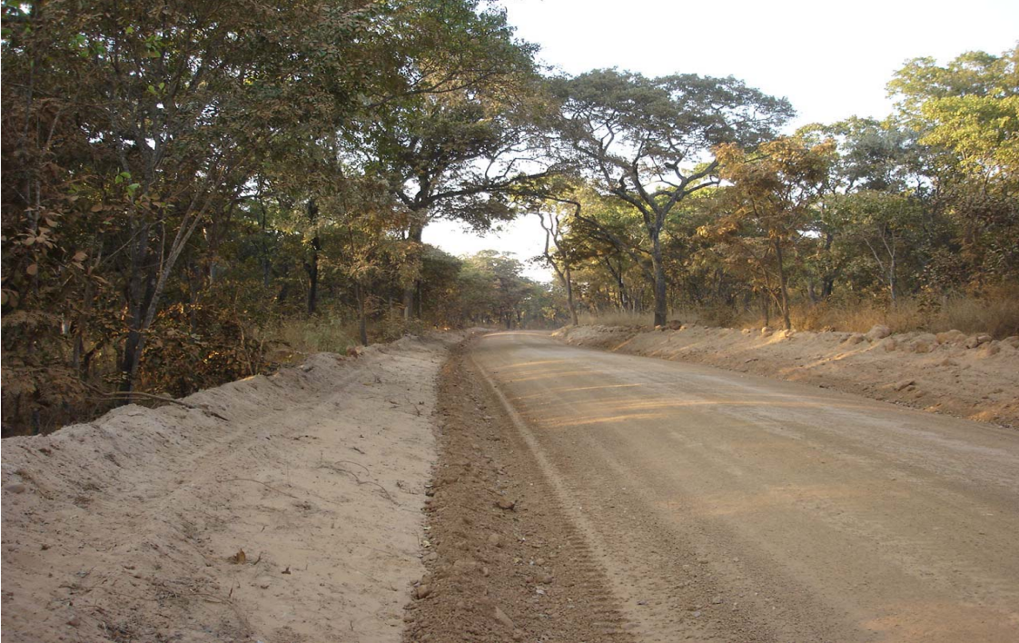
Figure 5: Road Construction in the Protected Area
