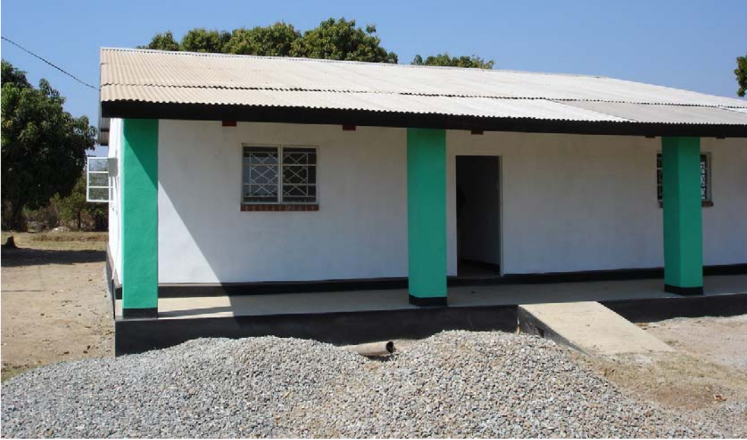
Figure 4: Clinic Under Construction
