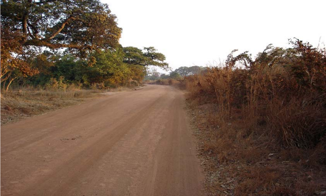
Figure 6: Part of the Road in Chief Nkana's Village
