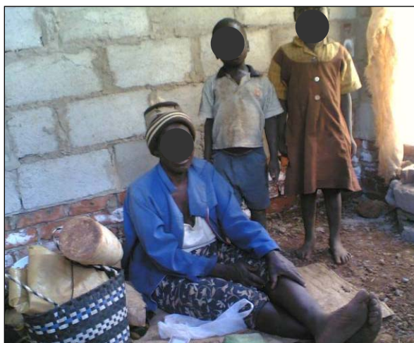
This family was moved into this clearly unfinished Operation Garikai/Hlalani Kuhle house at Hatcliffe in December 2005, shortly before the visit of Jan Egeland. © AI 2006
