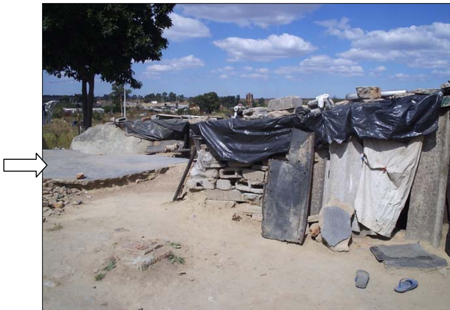
IDP campsite, Harare. Approximately 150 households were living on this site in May 2006 and had been living like this since their brick houses were demolished during Operation Murambatsvina. The foundation slab of one brick house can clearly be seen on left of photo (see arrow). © AI 2006
