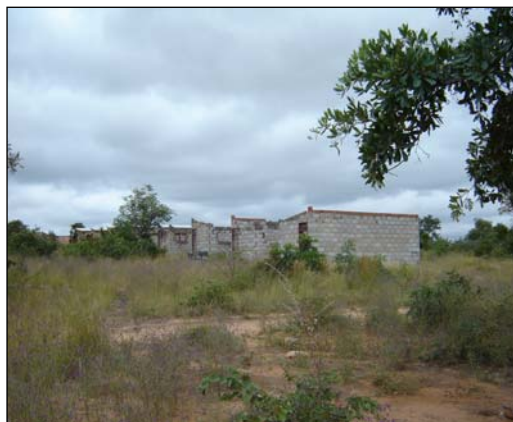
Cowdray Park Operation Garikai/Hlalani Kuhle houses in April 2006 (unfinished). © AI 2006
