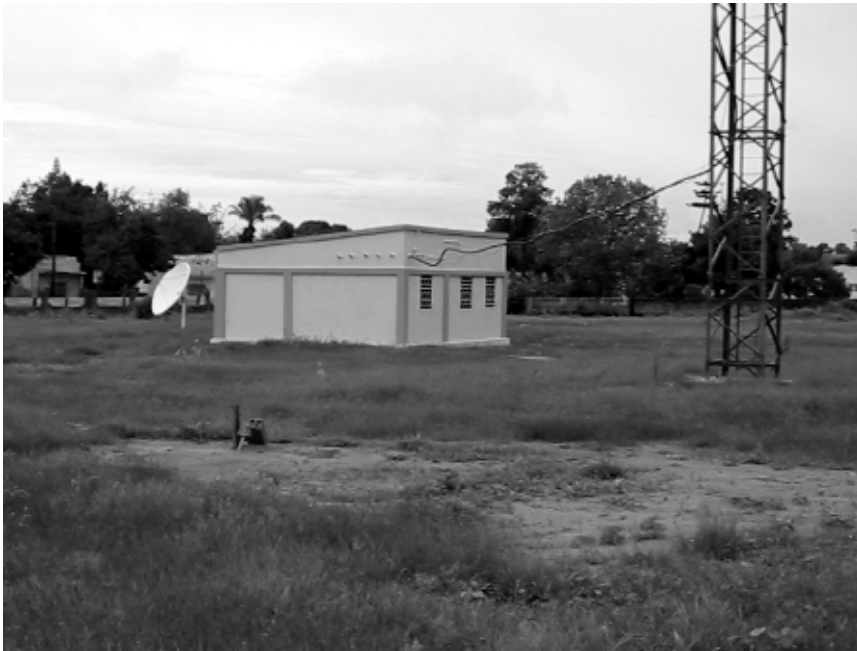
Rádio Ecclésia FM repeater station in Huambo, with satellite receiving dish linked to FM transmitter tower.
